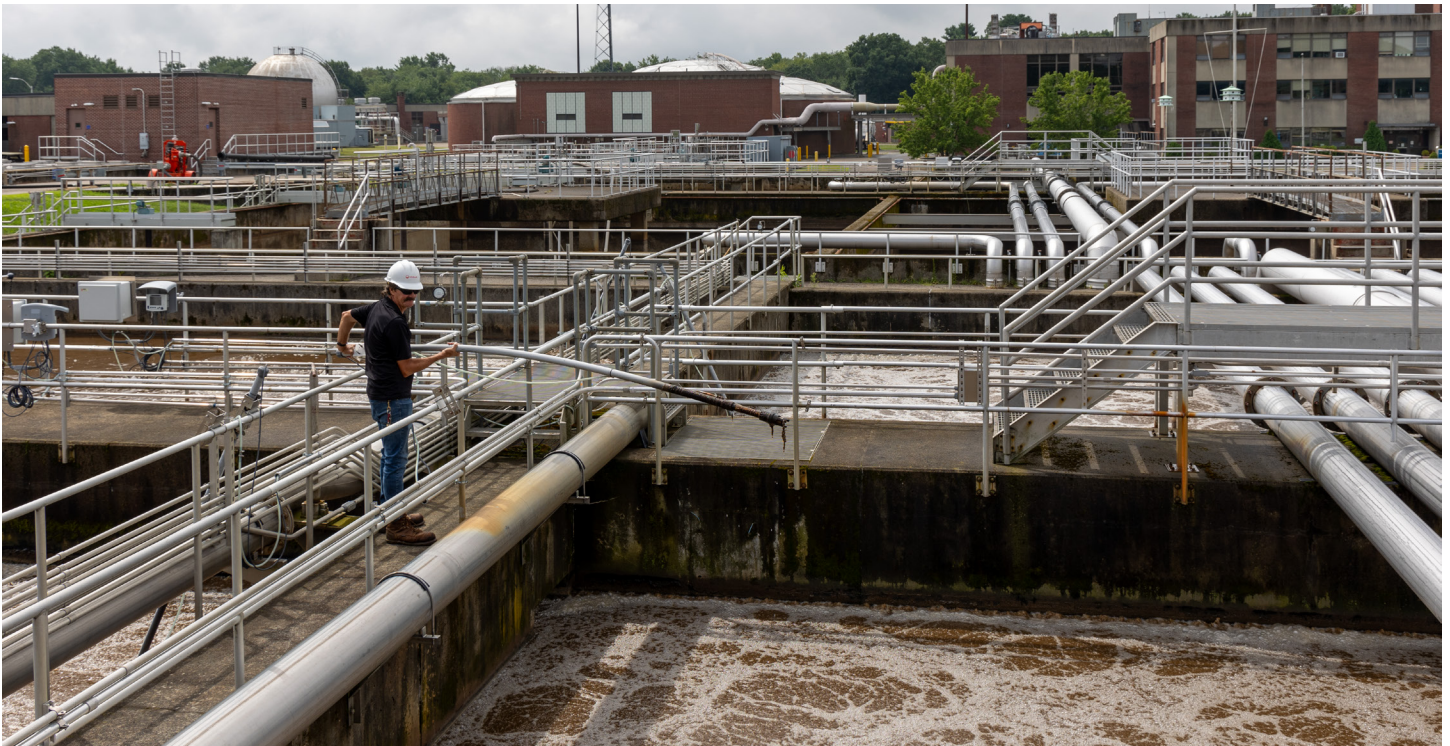
John Downey performing maintenance on the AmmoLyt ammonium ISE sensor in the North basins
